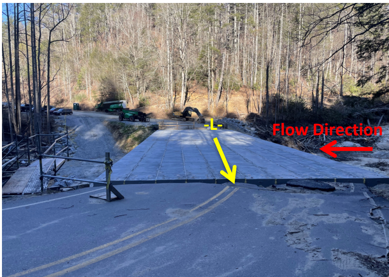
View at existing bridge location looking northwest.
