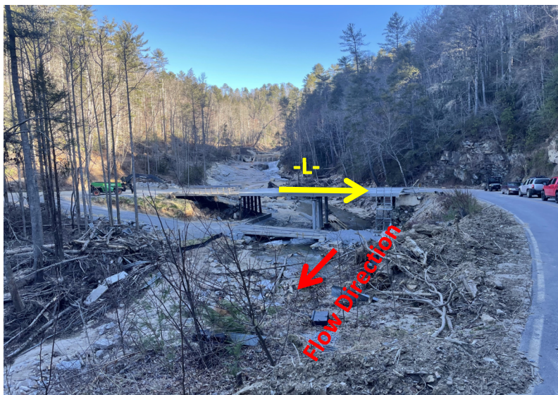
View of existing bridge location looking north.
